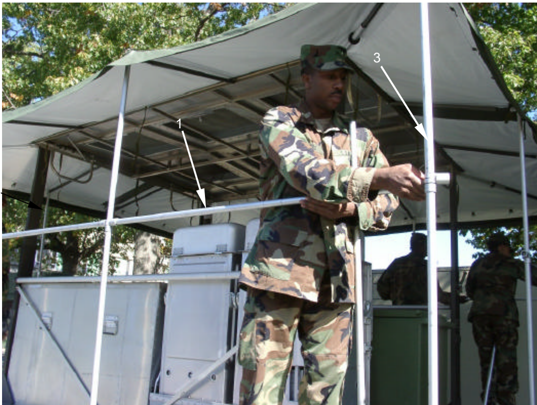
Insert handrails (1) into sockets (2) on tent poles (3) at sides and ends, allowing openings for entry and exit.
