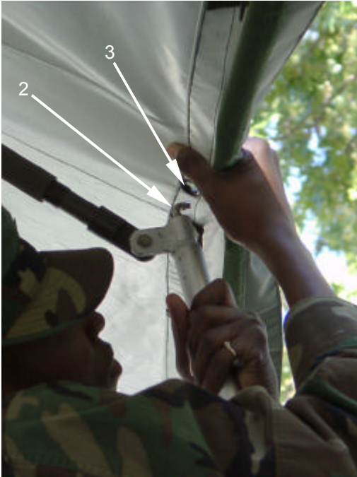
Insert handrails (1) into sockets (2) on tent poles (3) at sides and ends, allowing openings for entry and exit.
